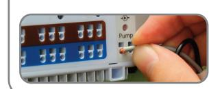
10 Push in the Boiler wires at the bottom
